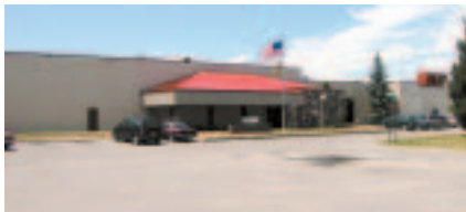
Parker Engineered Seals Division Headquarters - Syracuse, IN
